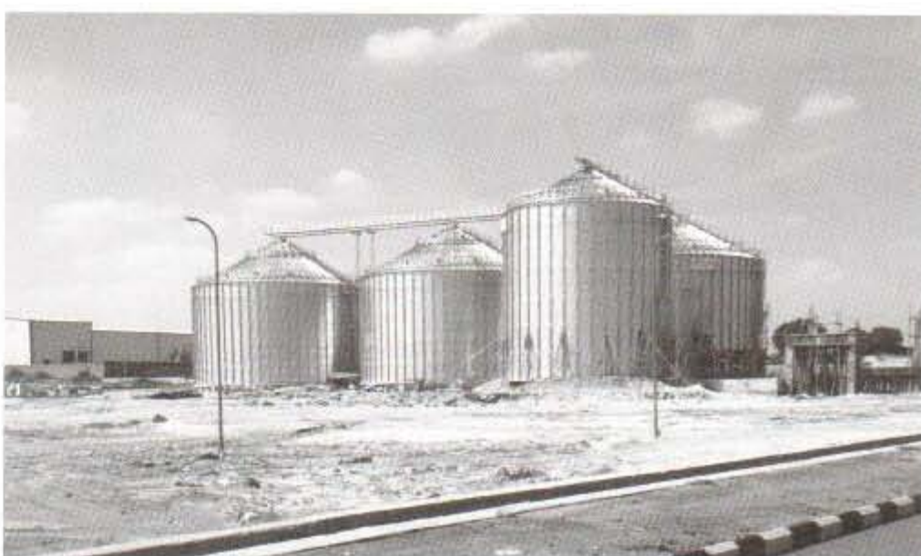
Silos at Integrated Food Park Private Limited in Tumkur, Karnataka.
